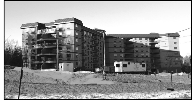
TRR photo by Fritz Mayer
